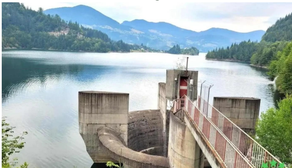
Barajul colibița colibița
