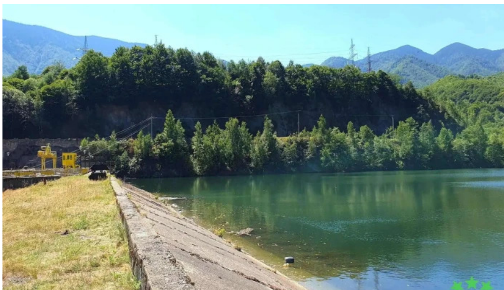
Barajul malaia pod
