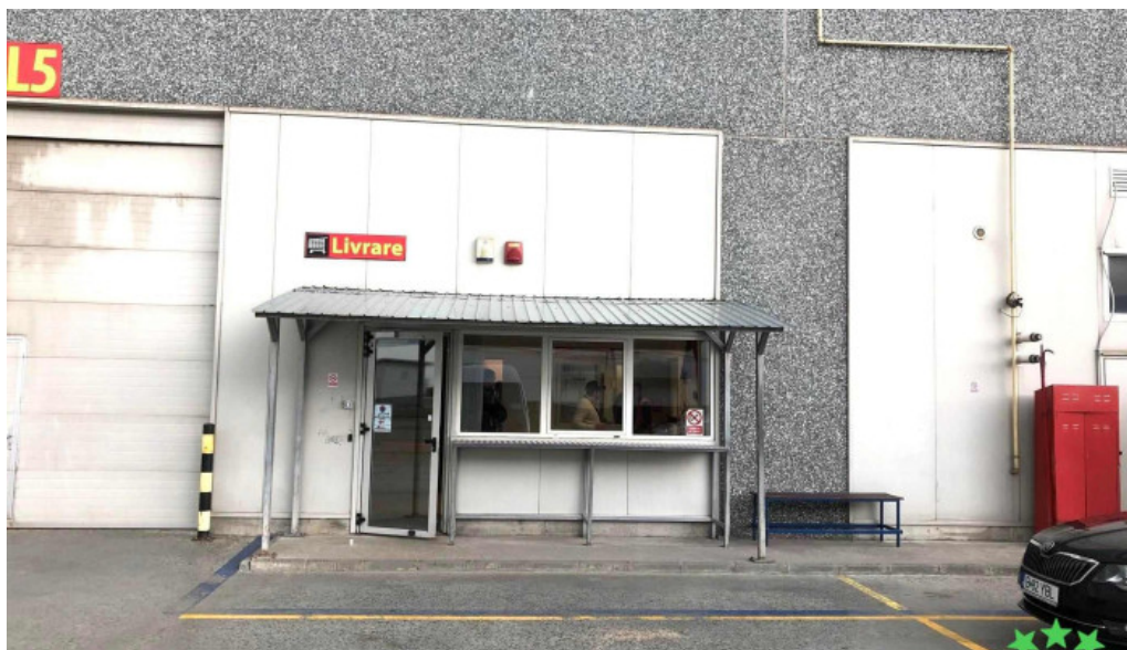
Augsburg international depozit central rima exterior
