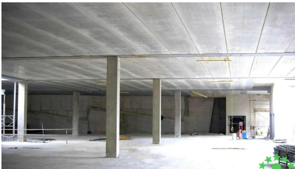
Peikko romania srl beton
