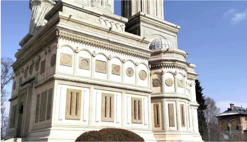
Next maintenance unde
